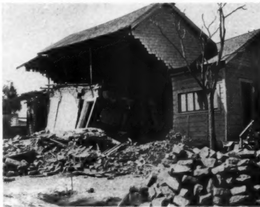
FIG. 12. SHOWING DESTRUCTION OF ONE OF THE OLDER ADOBES
